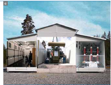
5 A MALTE prefabricated substation: old substation a , new substation b and interior of the new substation with a power transformer in the middle, high-voltage to the right, and medium-voltage and secondary equipment on the left c
