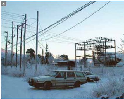
5 A MALTE prefabricated substation: old substation a , new substation b and interior of the new substation with a power transformer in the middle, high-voltage to the right, and medium-voltage and secondary equipment on the left c
